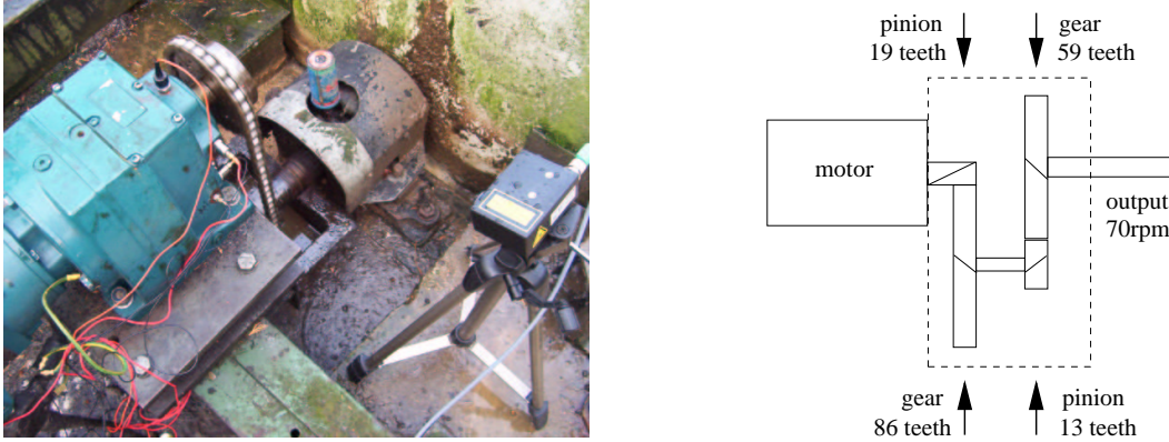
Fig. 2. Two-stage helical reduction gearbox used in a wastewater treatment site (left) and simple schematic (right).
