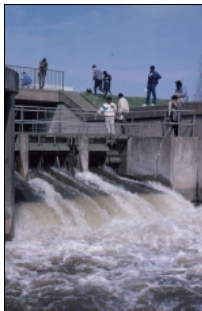
Figure 2.6 Neyrpic gate at Denver Sluice. Controlled rate of discharge (Photo T.M. Hess)
