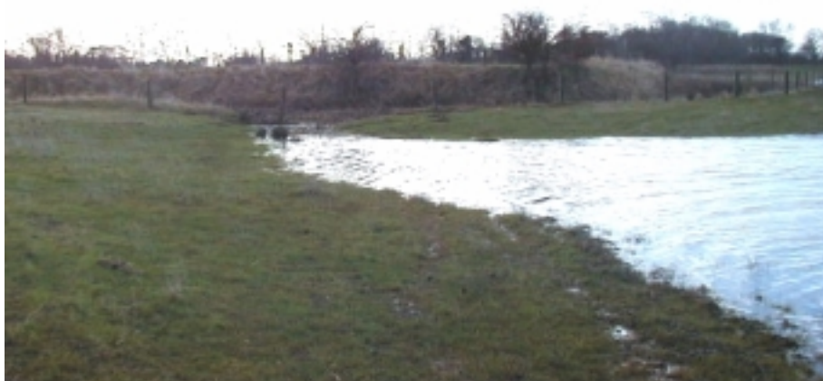
Fig A4.17 The main inflow and outflow point, a breach in the banks.
