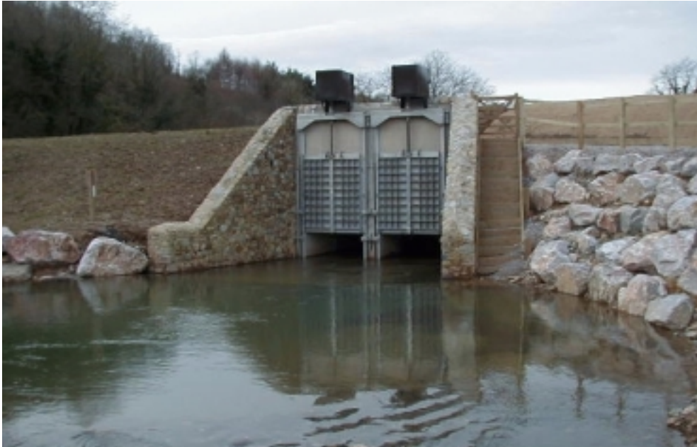
Figure A4.20. Sluice gates on the down stream side of the dam. In the foreground is a specially created pool for fish. Note how the dam structure has been naturalised as much as possible, and incorporates nesting facilities for dipper.
