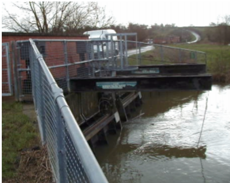
Figure A4.8 The non-return valve controlling the outflow from the River Chelt into the River Severn.
