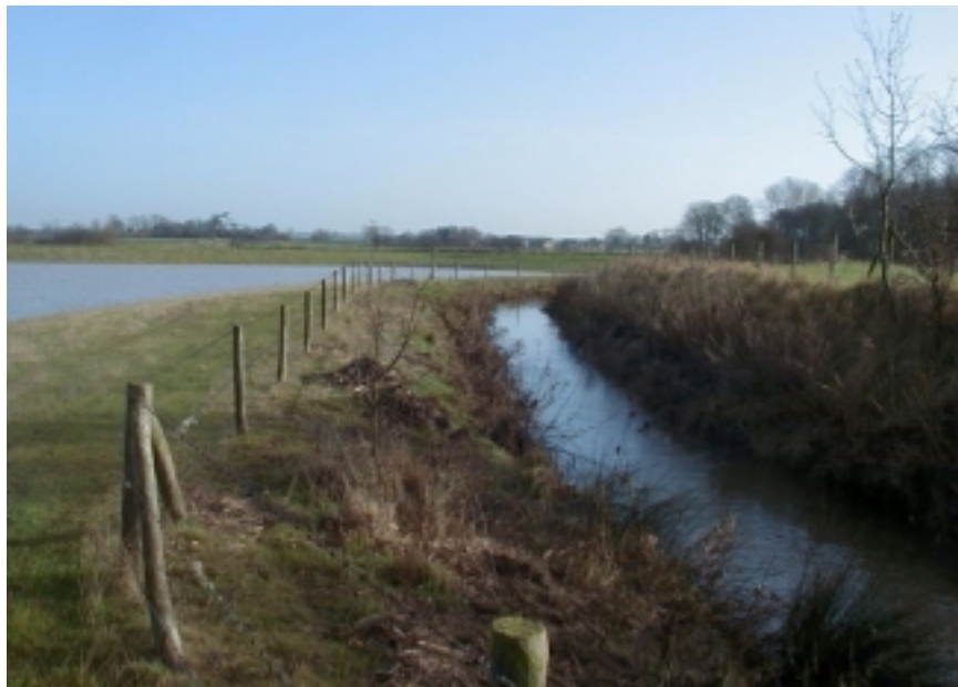
Fig A4.15 Long Eau flanked by old engineered bank (right) and the lowered re-profiled bank (left).
