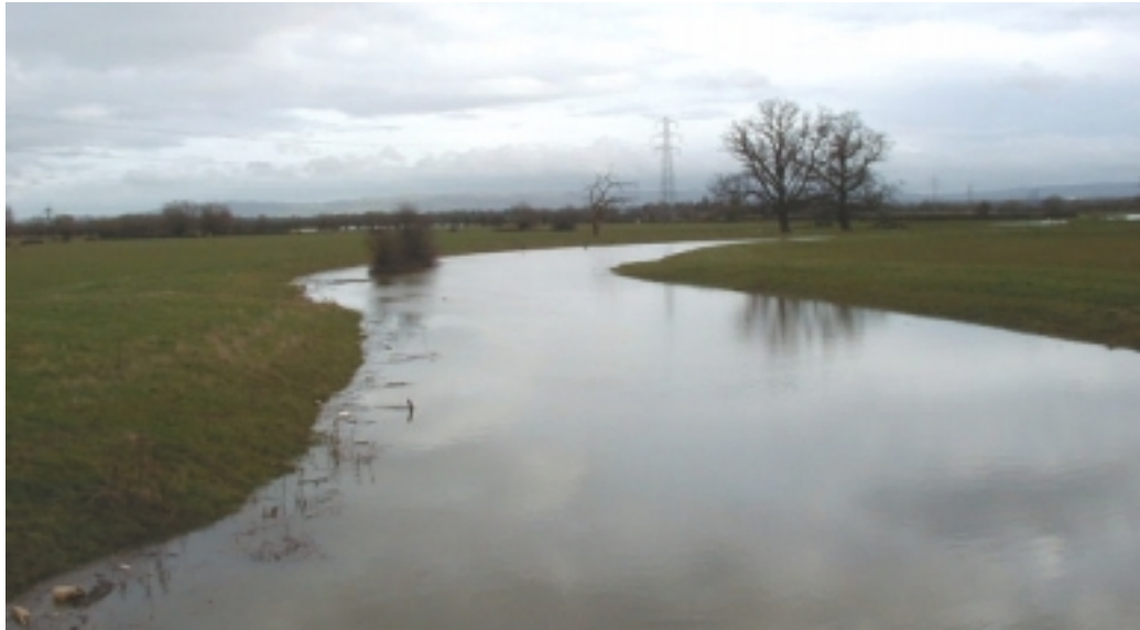
Figure A4.7 River Chelt with small embankments providing protection of grazing land against the annual flood.
