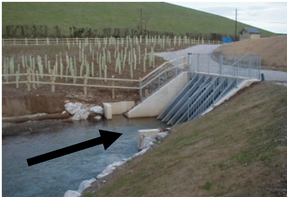
Figure A4.21. Upstream side of the dam includes the culvert structure. Note the newly planted broad leaf trees in the background.
