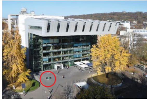
Fig. 12. The SuperC of the RWTH Aachen University, Germany g with borehole cover in the red circle [28].
