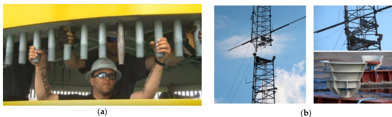
Figure 1. Examples of mechanical guidance systems: (a) Current use of guide pins; (b) Guide cones for human-free met mast installation [4].
