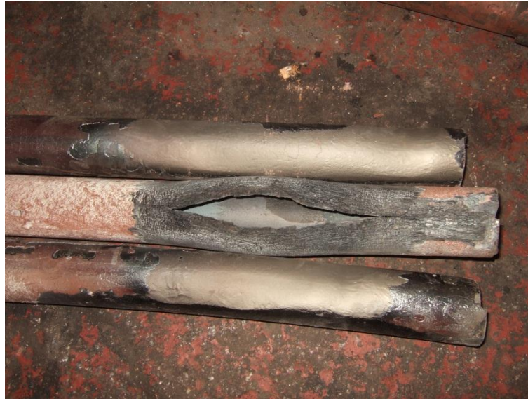
Figure 1.2 Superheater tube from a utility boiler failed by creep
