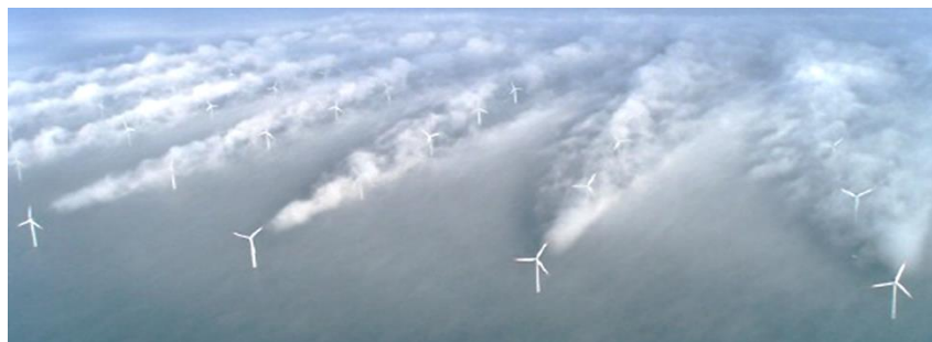
Figure 1-1 Conventional wind farm of horizontal axis wind turbine
