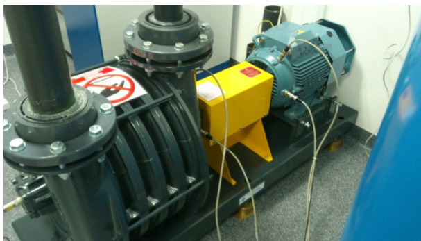
Fig. 109: Arrangement Motor-Compressor
