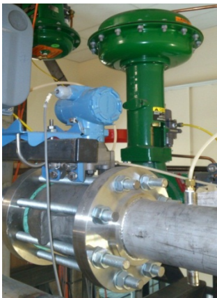
Fig. 15: Top separator input valve VC404
