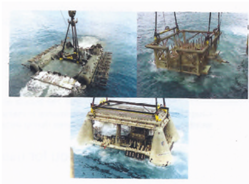
Figure 2-8 Examples of Subsea structure in the splash zone
