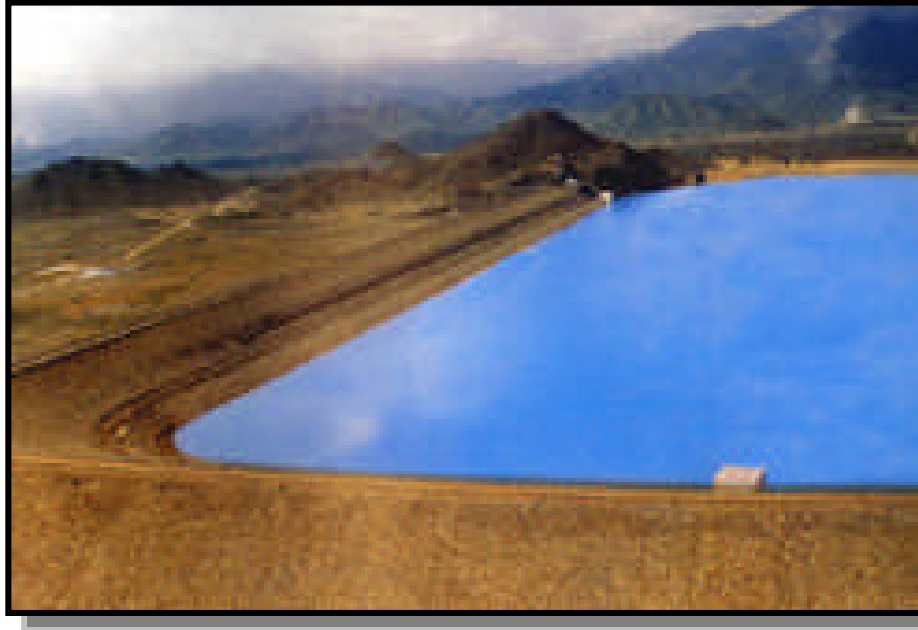
Figure 3.19 Wadi Ham dam reservoir filled with flood water (Source: www.uae.gov.ae/maf ).
