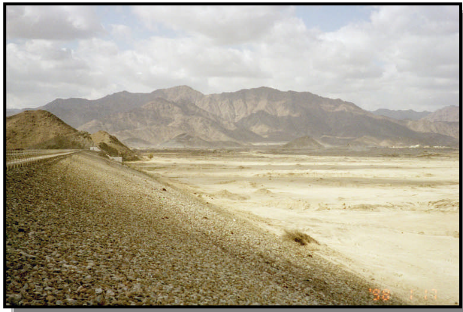
Figure 3.18 General view of Wadi Ham dam reservoir.
