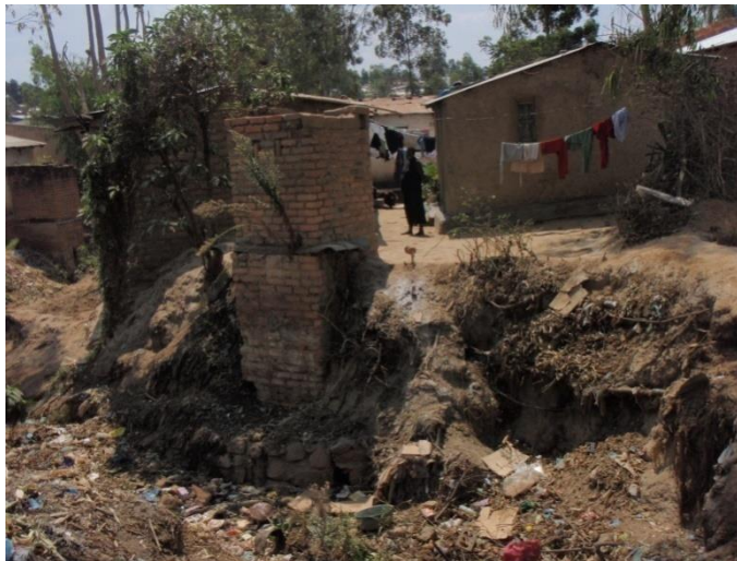
Figure 11: Latrine that backs directly on to the river
