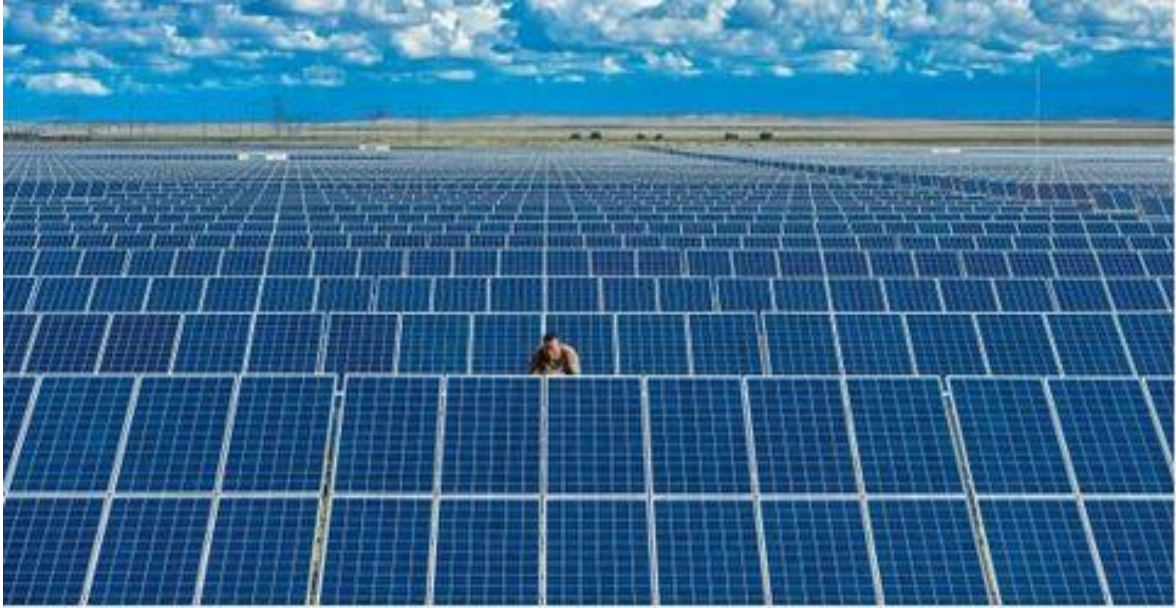
Figure 2-7: 175 MW Solar PV Farm in South Africa ( The largest Solar Farm in the Southern hemisphere is located in Central South Africa, 2017 )
