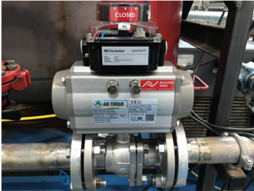
Figure A.2-2 Pneumatic safety valve
