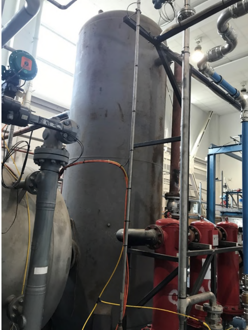
Figure A.1-2 Air receiver (the long grey cylinder)
