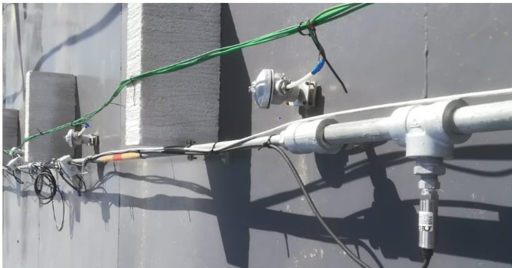
Figure 107 - Nitrogen distribution network
