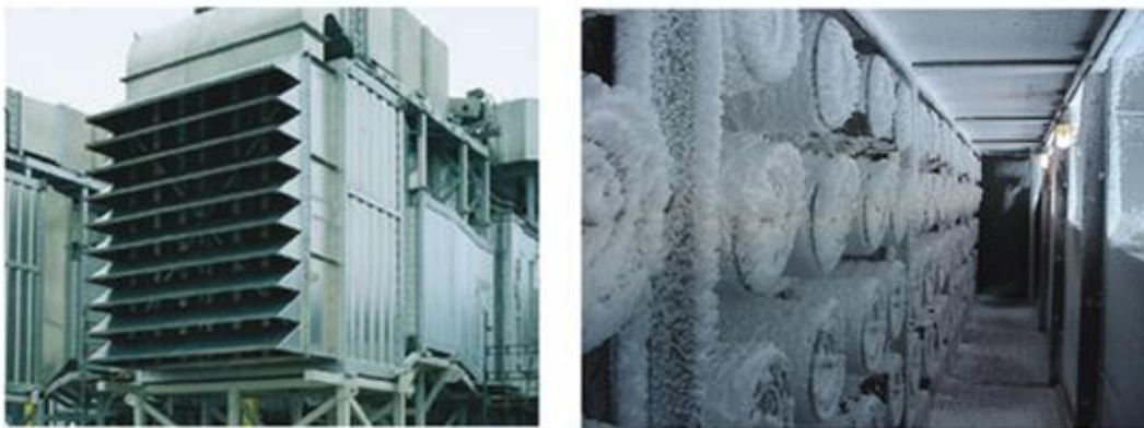
Figure 2-17 Example of weather hood (left) [70] and pulse cartridge filters on ice (right) [33]
