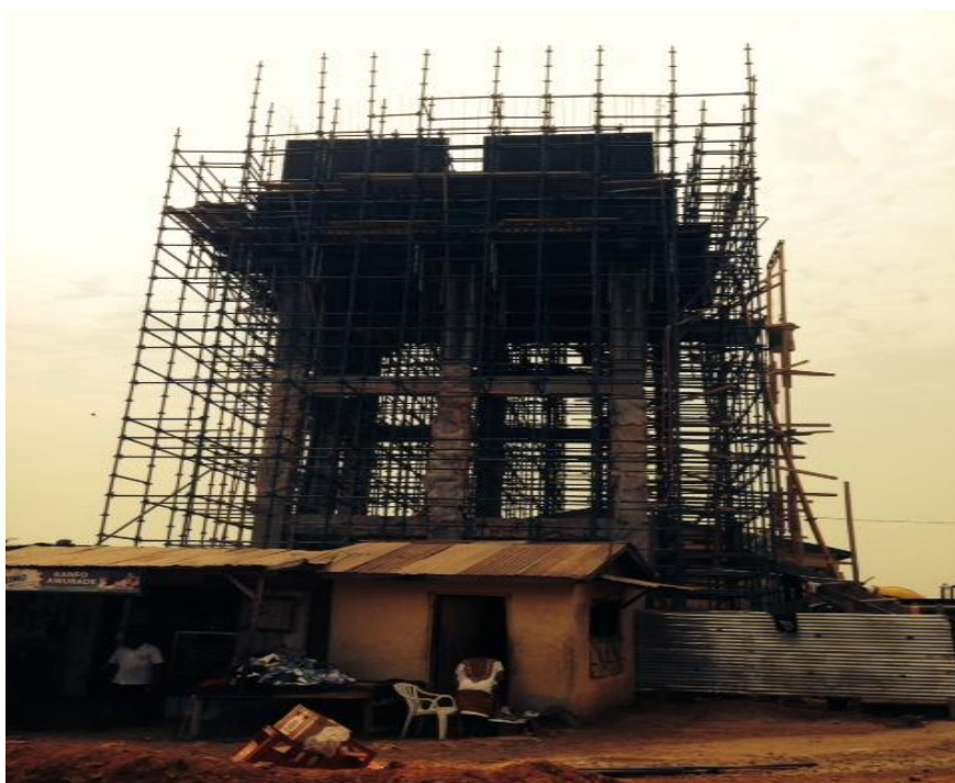
Figure 4-2 construction of an overhead tank
