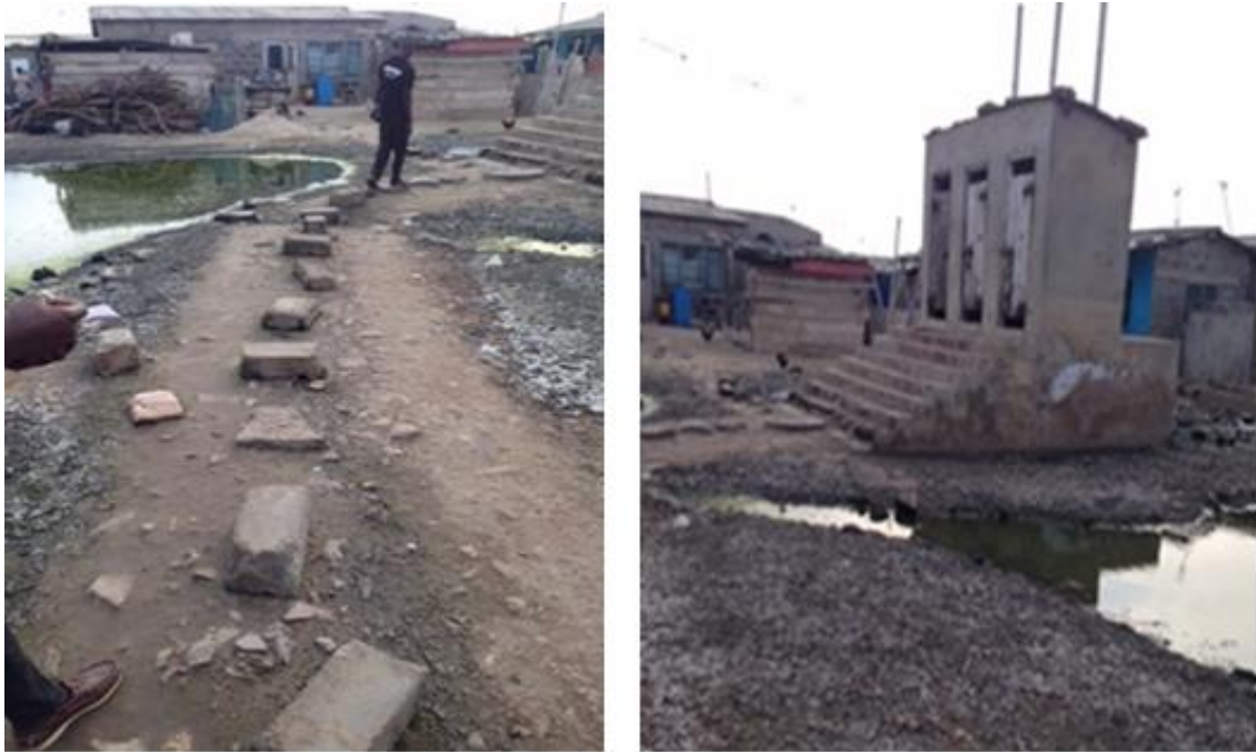
Figure 4-10 Toilet designed against flooding
