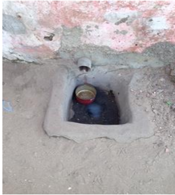
Figure 4-12 Grey water collected in containers
