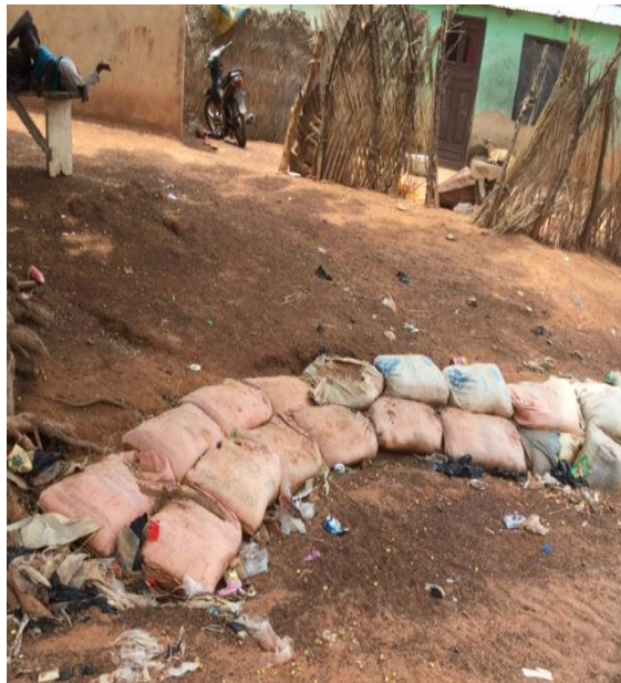
Figure 4-16 Sack filled with sand to divert runoff
