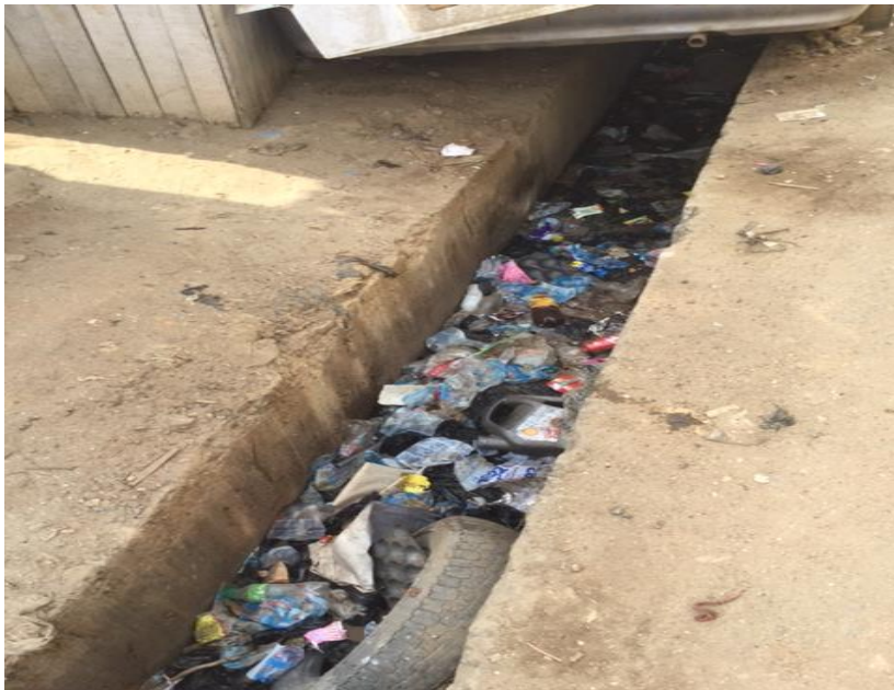
Figure 4-5 chocked drains in Glefe
