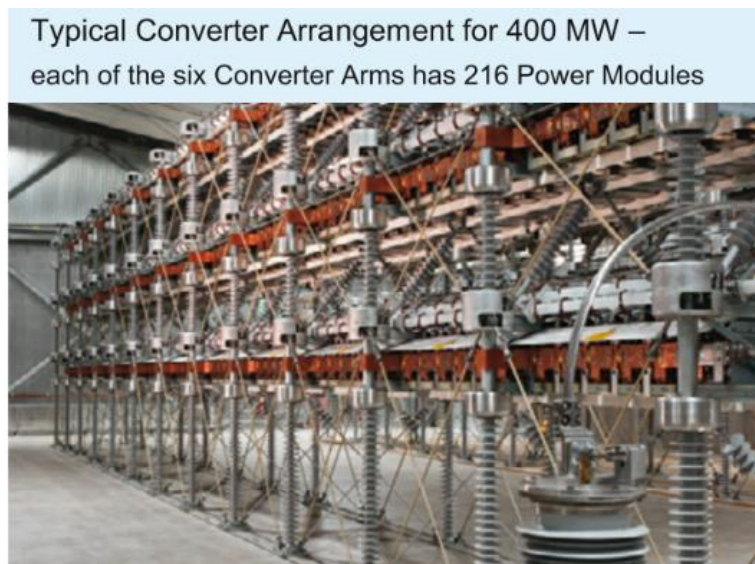
Figure 2-8 Voltage source converter [151]
