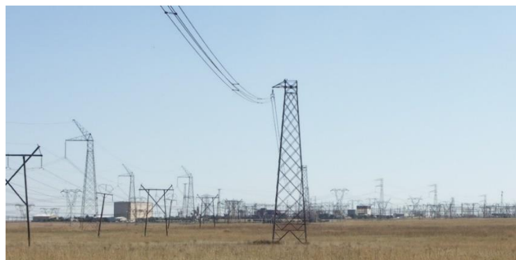
Figure 2-21 Apollo monopolar converter station [208]
