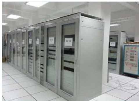
Figure 2-1 Integrated control system of Nan’ao Multiterminal VSC [130]
