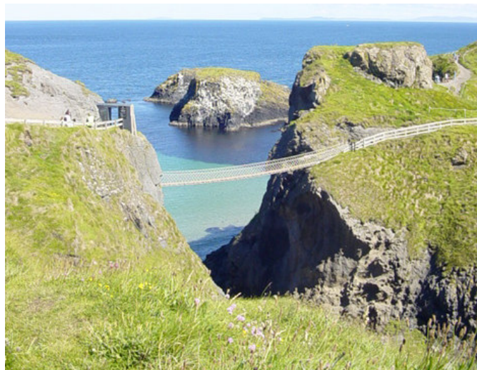
Figure 7-4 A catenary - the Carrick-a-Rede rope bridge
