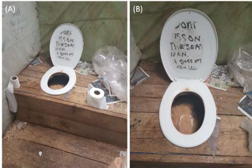
Figure 77 – (A) The toilet area and (B) the view inside of the UDDT at the eco-community (Tierney, R. 2017)
