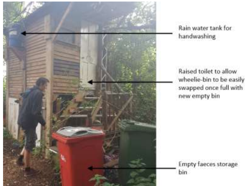
Figure 76 – One of the two raised toilets that the eco-community have built and use with one of the residents demonstrating storage and processing of the excreta (Tierney, R. 2017)
