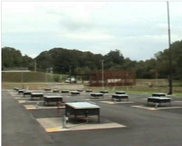
Figure 1-1 Removable metal trays on concrete pads at an installation used for the burning of explosives [1]
