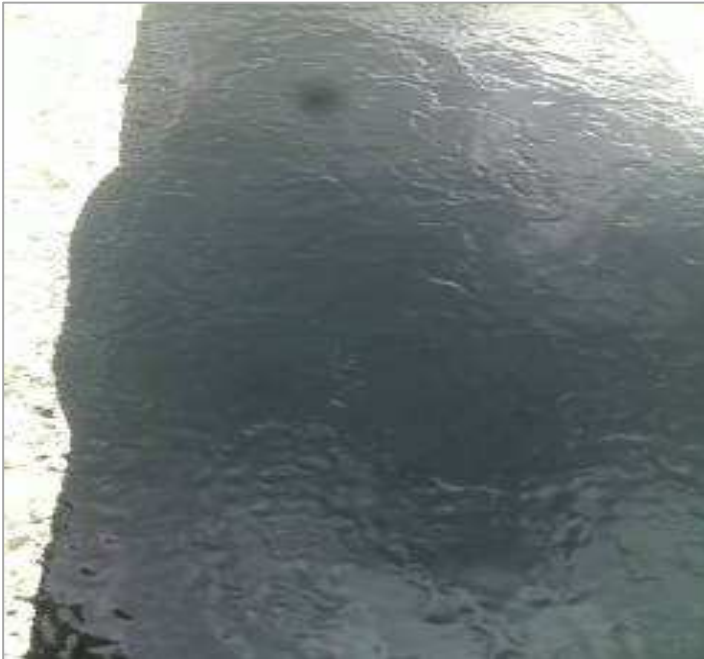
Fig. 6-8. Cold asphalt, treated smooth surface
