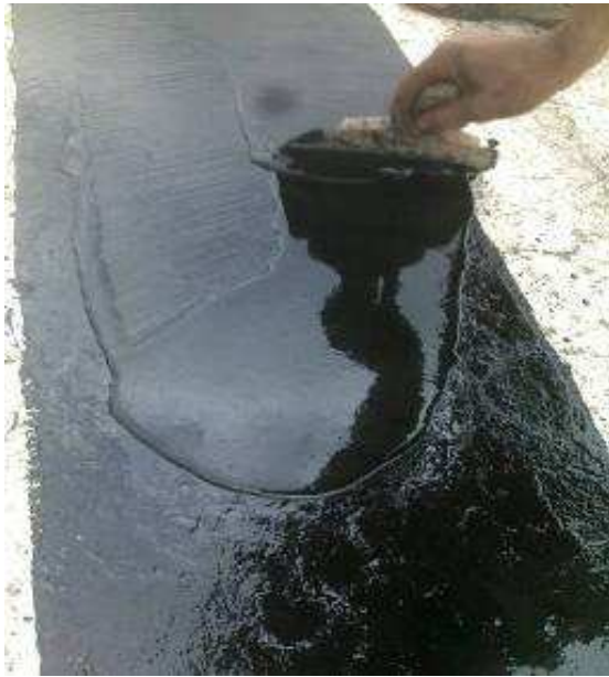
Fig. 6-4. Levelling of asphalt slurry
