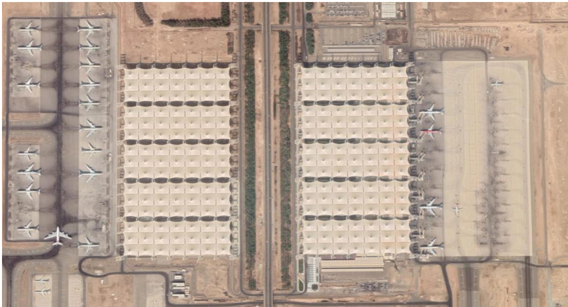
Figure 2-4 HT at Jeddah Airport - top view
