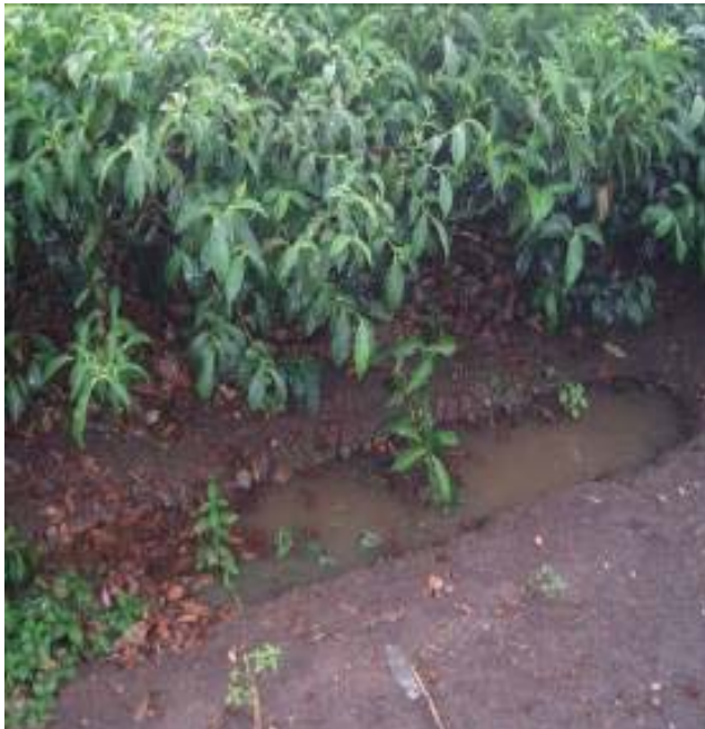
Figure 8. Example of a lock and spill drain on the KGTF Ntungamo estate.
