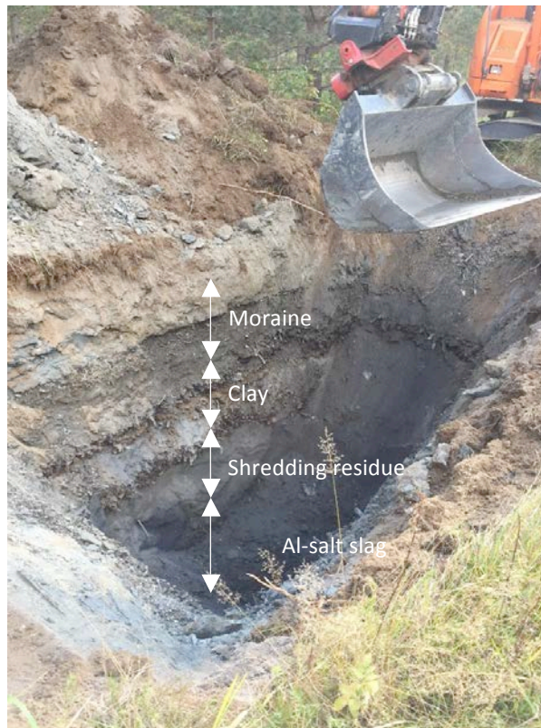
Figure 4: Landfill layers at the Vierumäki industrial landfill.
