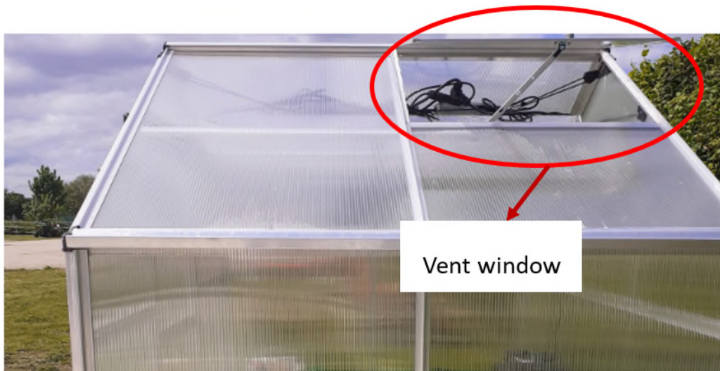
Figure 6.4 Natural ventilation
