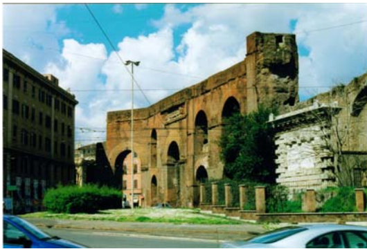
Brick faced concrete, Nero's branch, Rome
