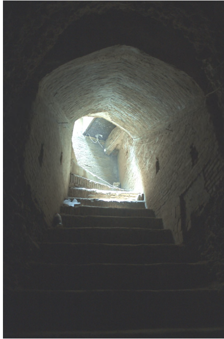
Figure 6. Stairs view from the bottom
