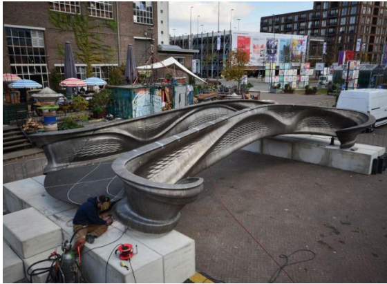
Figure 1. MX3D bridge (Liwanag, 2020).
