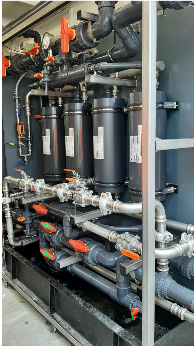
Figure E-2 Demonstration-scale degassing system for the removal of dissolved methane.
