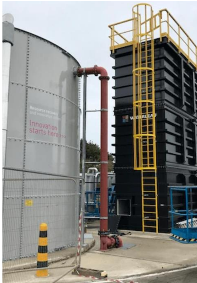
Figure C-1 Demonstration-scale UASB reactor (in black).
