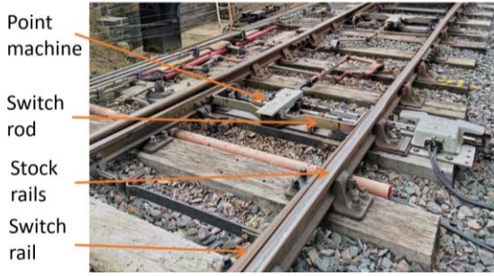
Fig. 5. Basic components of a switches and crossings
