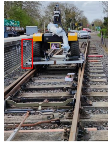
Fig. 4. Congested space between the track and platform
