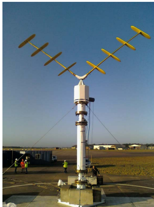
Figure 1. Prototype of original NOVA V-VAWT concept.
