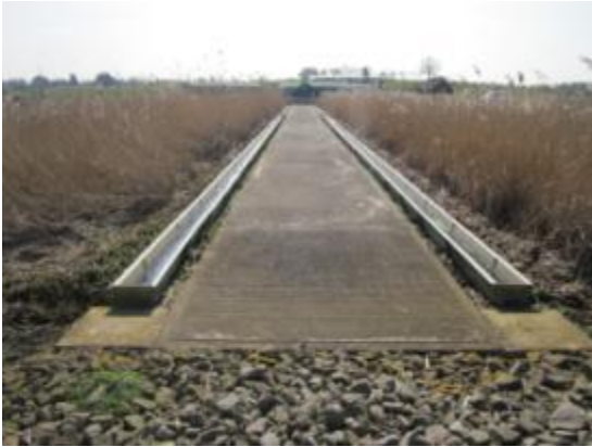
Image 1. Inlet channels of the reed beds
