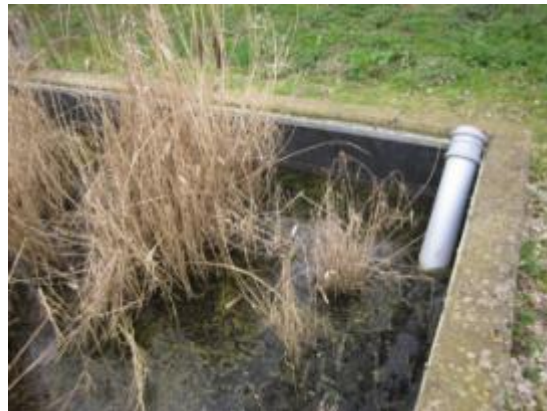
Image 4. Flooded outlet zone of the reed bed
