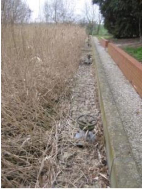
Image 1. Inlet zone of the reed bed.
