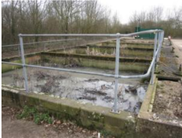
Image 7. Old storm tanks used as holding tank
