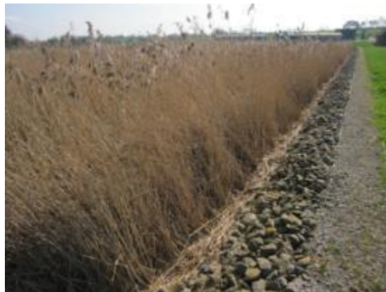
Image 4. View of the reed bed from the outlet zone
