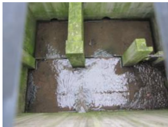
Image 6. Splitting chamber
