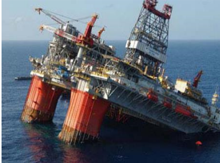
Figure 11 A semi-sub rig collapses in ultra-deepwaters (UDW Report 2005).
