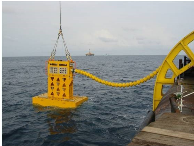
Figure 24 Subsea equipment deployment
