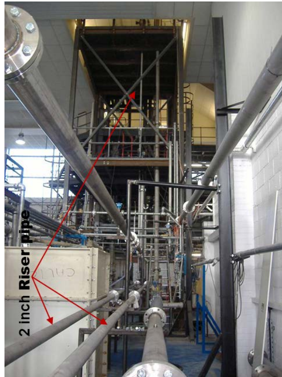
Figure 3-3: Actual picture of the 52 mm riser rig in the flow laboratory
