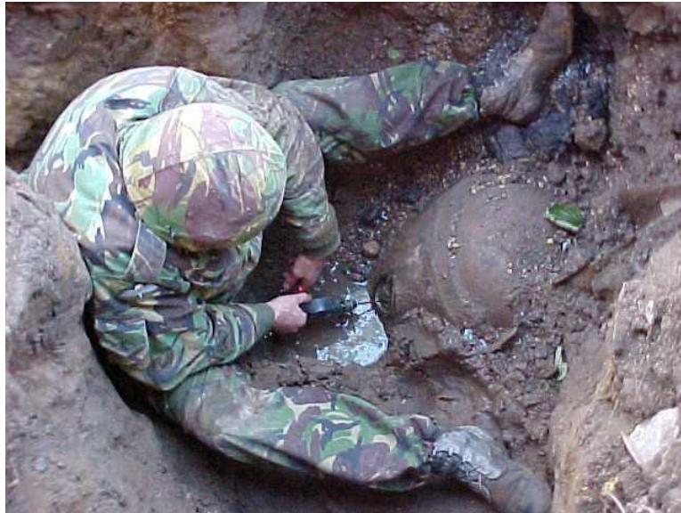
Figure 2.20: A Royal Engineer defuses a WWII bomb in Sunderland, UK after access has been excavated (MOD, 2002)
