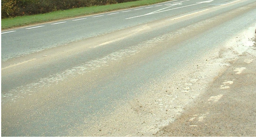
Figure 9 Contamination of a public road ~200 m from the entrance to a quarry that has a ~ 0.8 km access road. Vehicles were not being cleaned at the time the photo was taken.
