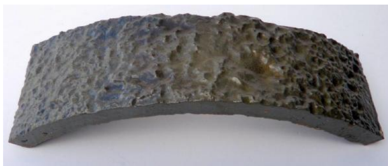
Figure 5 Characteristic pitting in water mains pipe due to soil-water corrosion. (S. Hallett)
