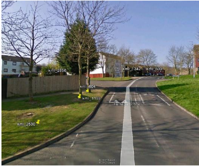
Figure 18 Example burst location proximal to road speed bumps, subject to potential vehicle loading from passing traffic.(Northampton, Google Street View)
