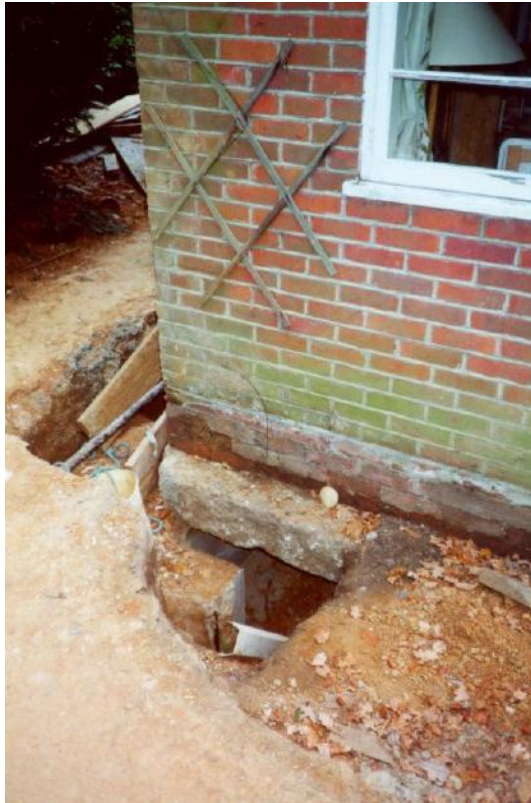
Figure 8 House underpinning necessitated by soil-related subsidence. (S. Hallett)
