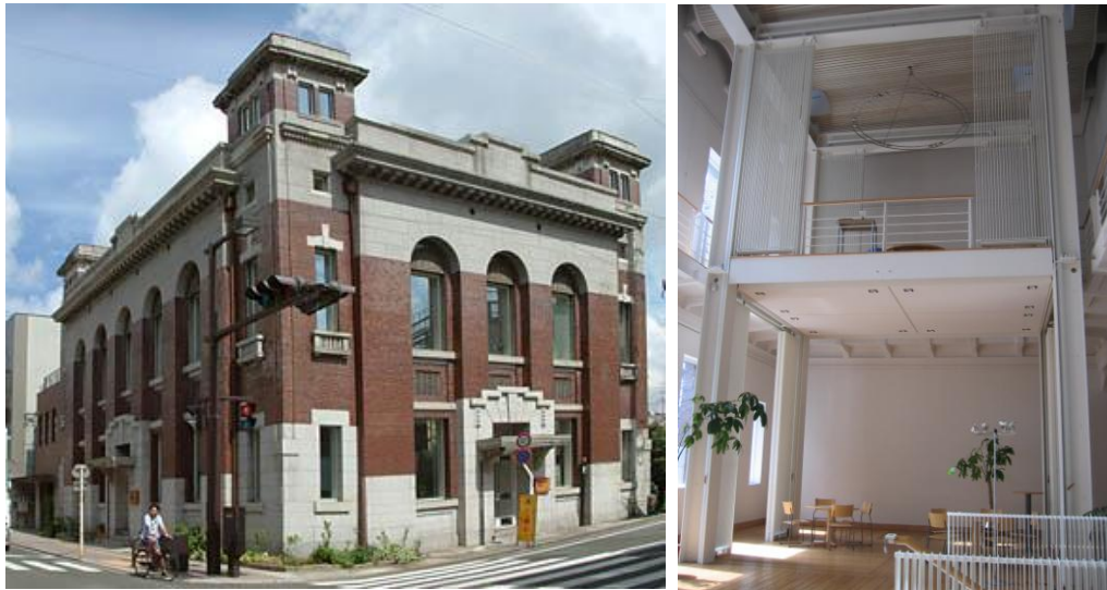
Figure 4.9. Photographs of the Orangeri building after refurbishment.
