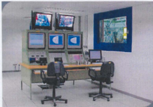
Figure 2.15: Modern Test Cell Control Room (Cell Aerospace Test Equipment)
