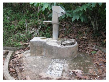
Figure 4: Broken and unused hand pump in the research area.
