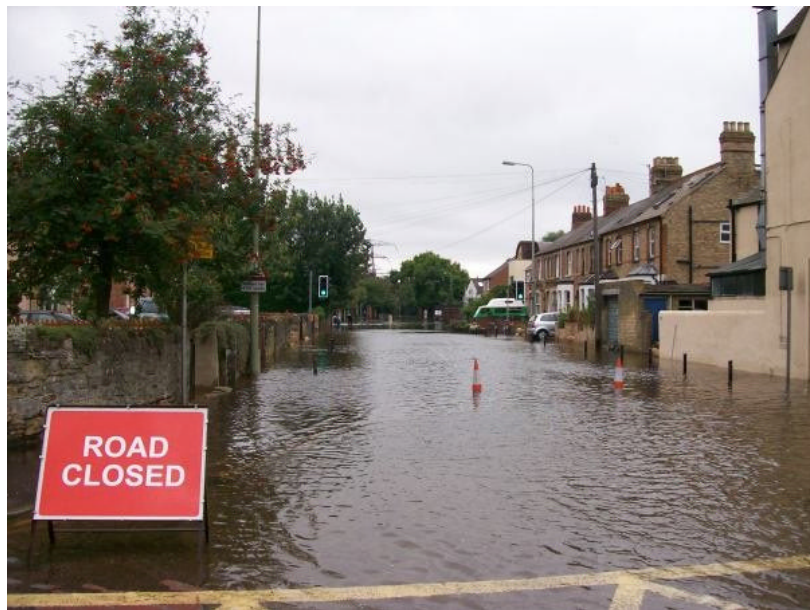
Figure 5.2: Flooding in an Oxfordshire street (Courtesy of A. Davies, 2007).
