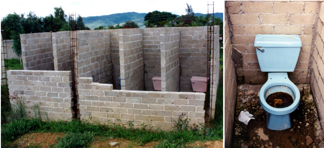
3 4 Figure 2. The 'new' toilets of Morelos primary school.
