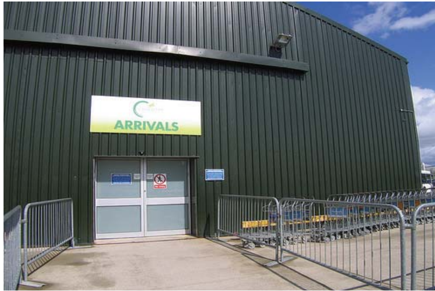
Figure 4.4 Arrival Area in Coventry Airport, UK (Source: Coventry Airport)
