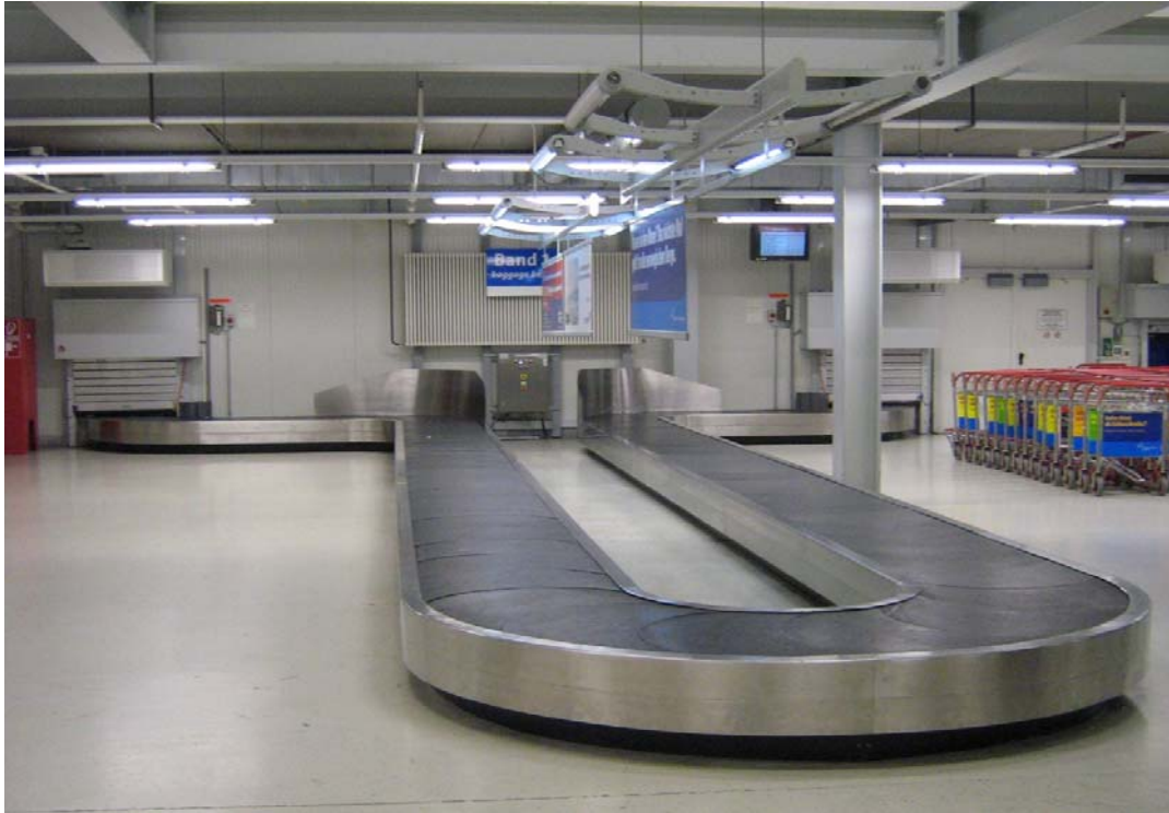
Figure 2.6 Baggage Handling Belts at Hahn Airport (Source: Hahn Airport)
