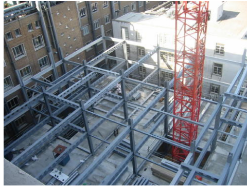
Figure 8: Steel Frame Multi Storey Office Block
