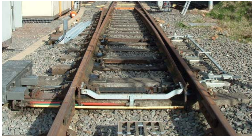
Figure 3: Full depth CV Railway Points
