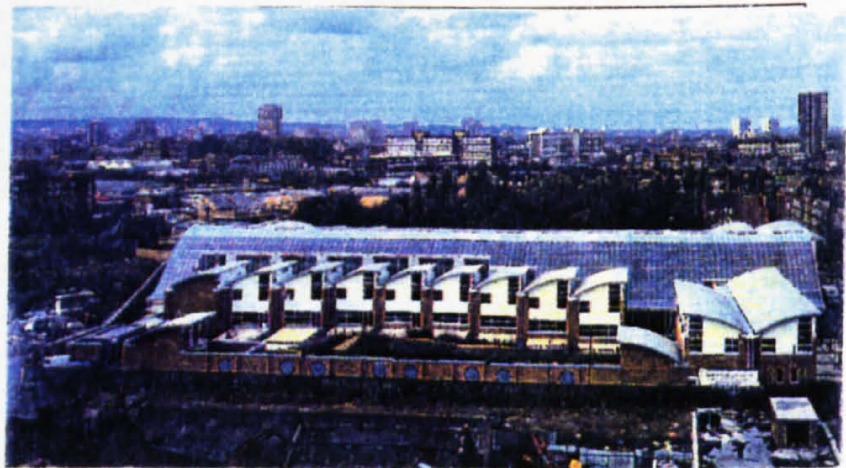
View from the south
