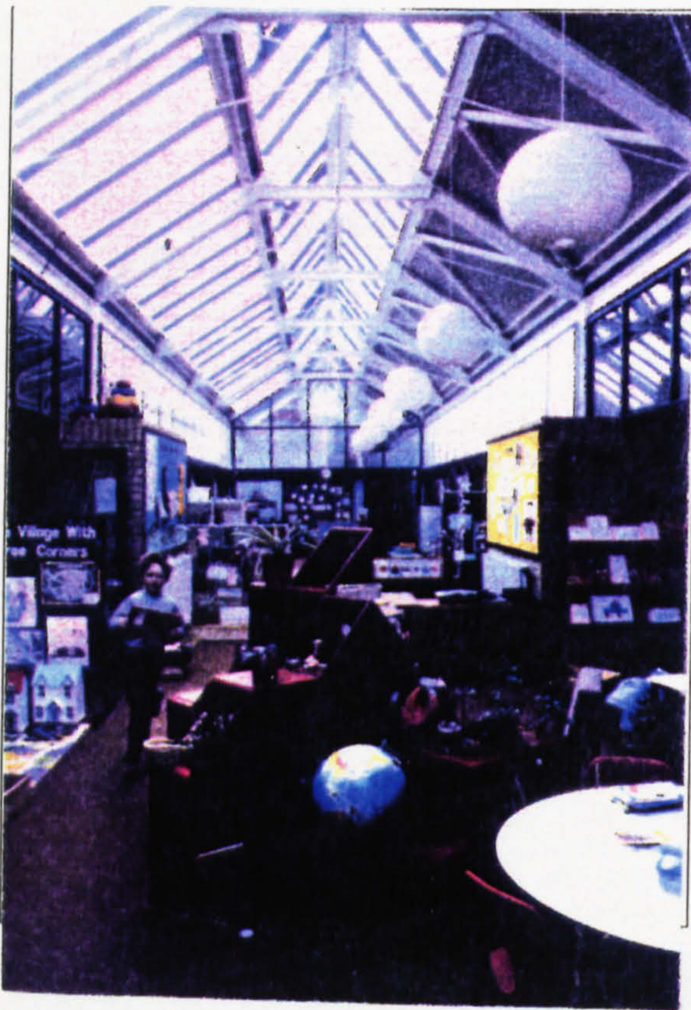
Interior of heated atrium. The opaque surface of the south facing roof prevents excessive solar gain
