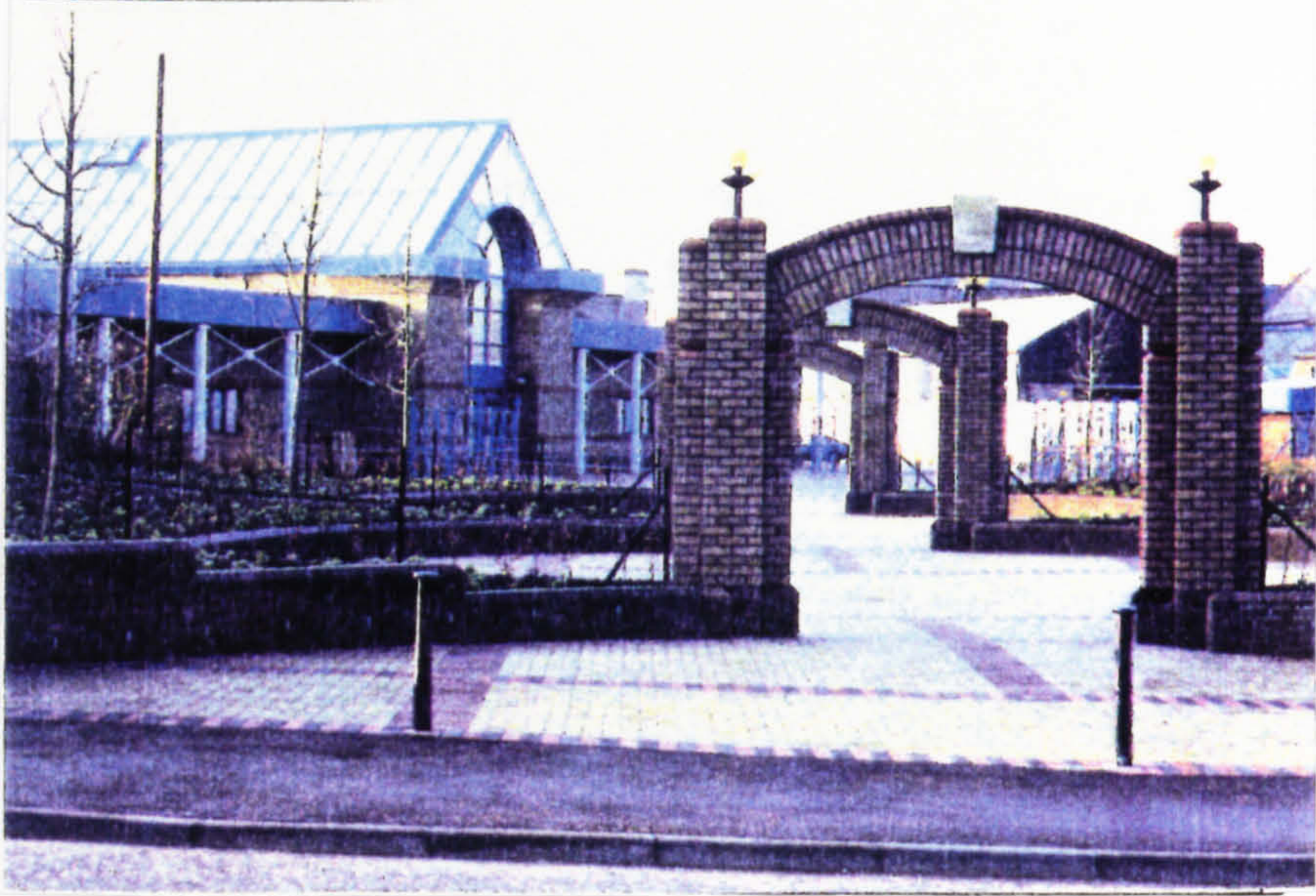
North Facade and main entrance from street
