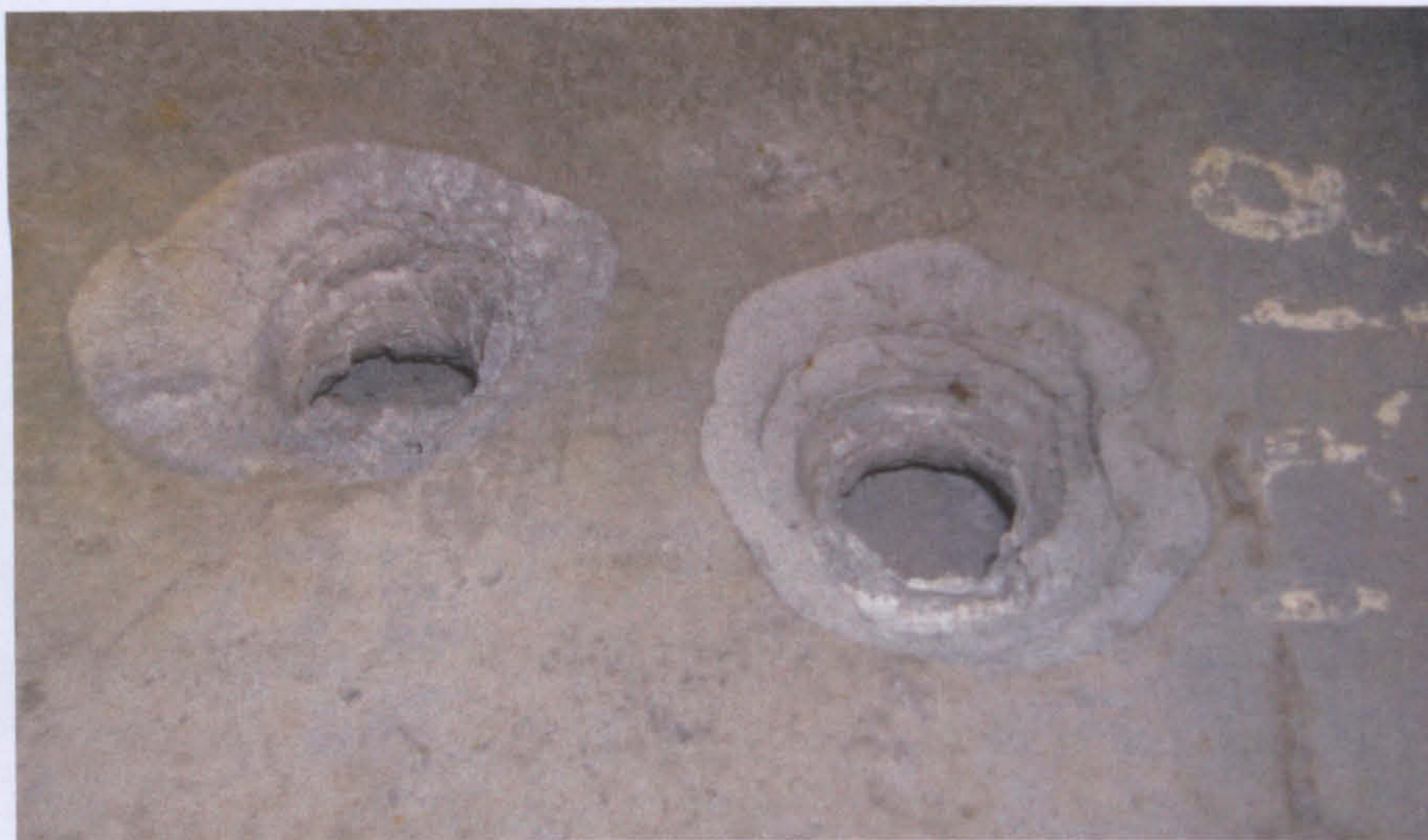
Image 6.1: spall of aluminium
