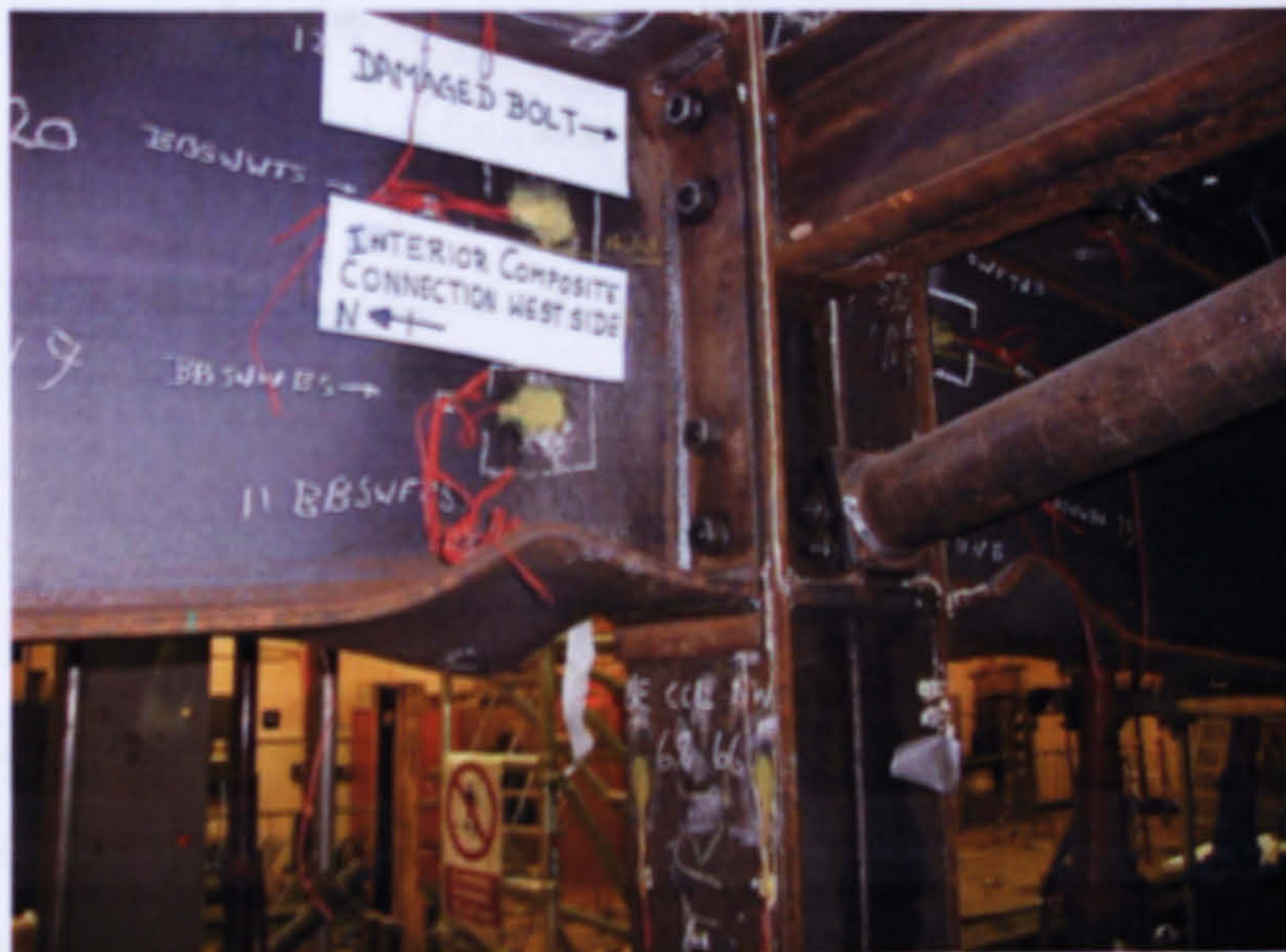
Figure 3-28. Interior composite connection (pin connection side) after test frame failure
