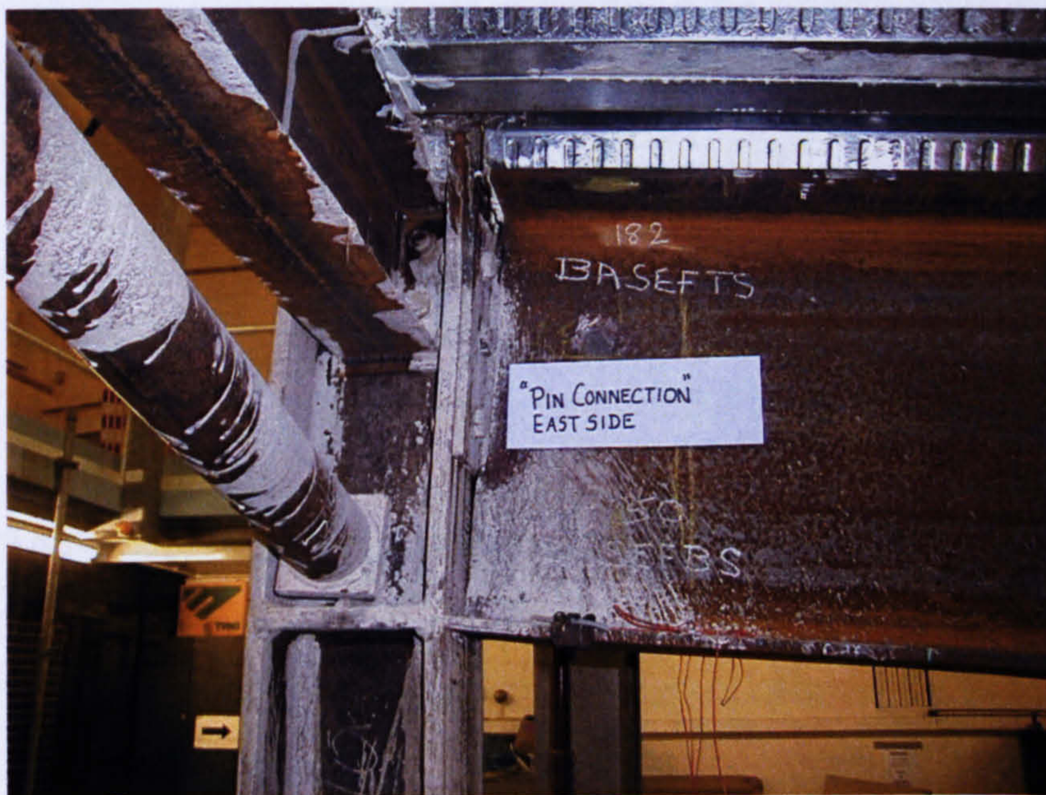
Figure 3-22. South side pin connection after test frame failure
