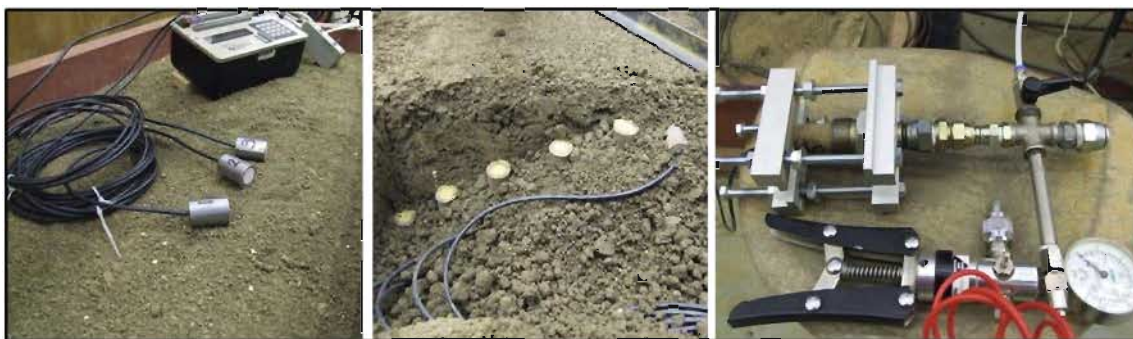
Figure 7.4 Sensors with Campbell micrologger (left), sensors buried (centre) and calibration airline (right).
