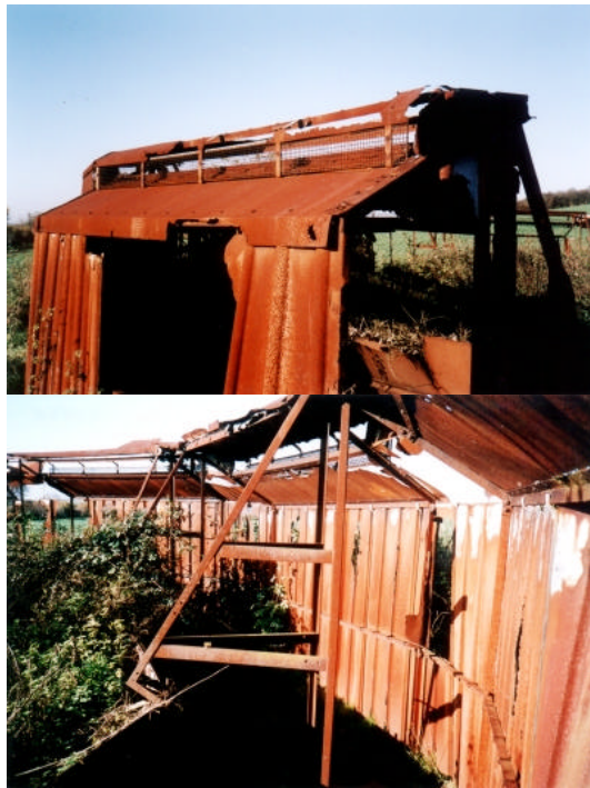
Fig 58 c,d. North Fambridge Silhouette site, detail of buildings. (Ibid.).
