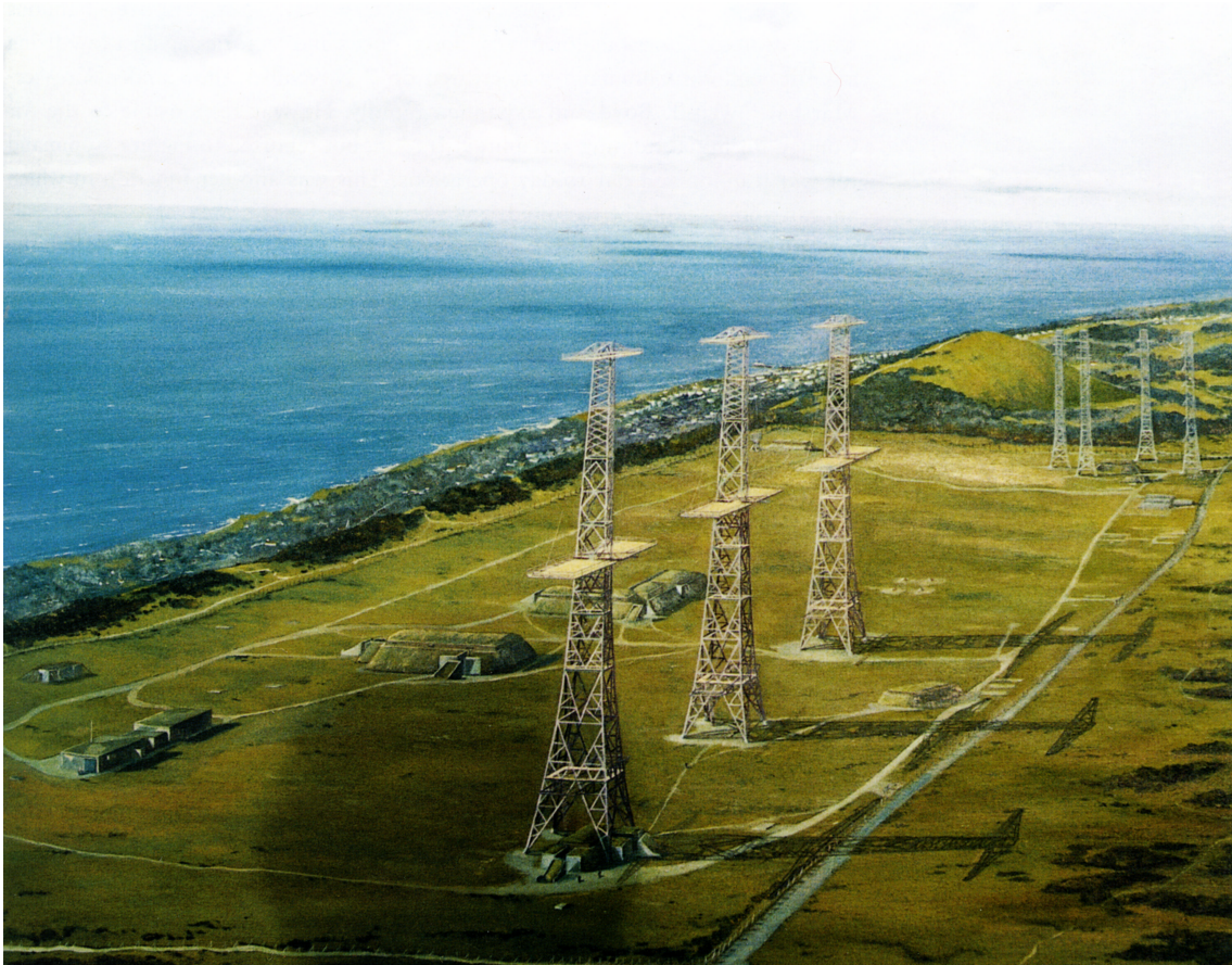
Fig 29. Ventnor Chain Home station. Apart from the fact that Ventnor was positioned above high cliffs, this picture of Ventnor is reasonably representative of the South Coast Chain Home stations. Ventnor was to be the most heavily bombed station in the battle of Britain. (“The Second Step – National Defence” by John Finch, Knowler Edmonds Collection).
