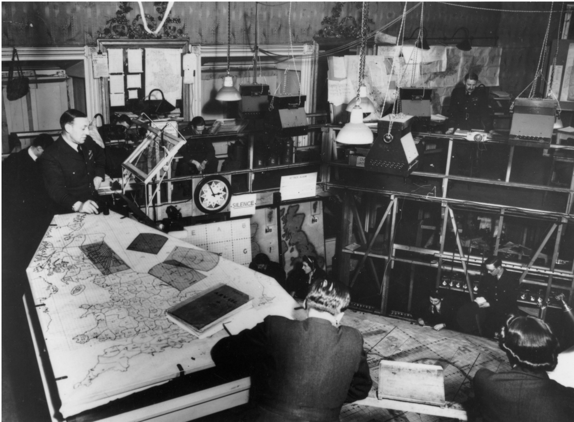
Fig 32. The earlier Operations Room, platform level, with the lower level map of Fig 31 at the lower right. The improvisation from the house's ballroom is clearly visible. (Peter Flint, op. cit. , Fig. 15/ Crown Copyright).
