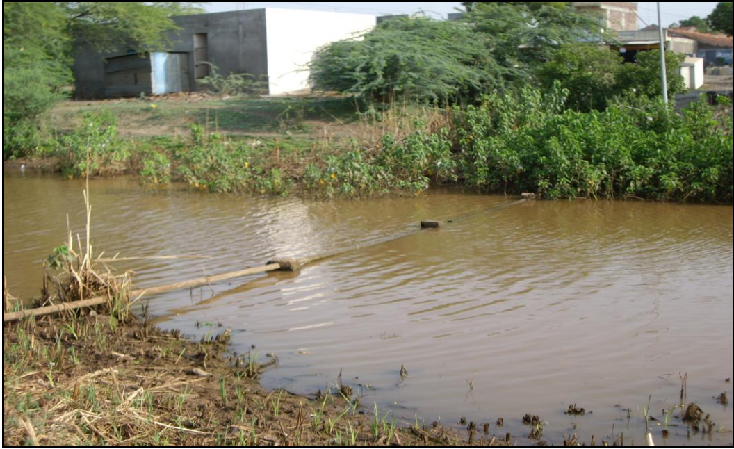
Plate 14: Partially submerged water pipe supplying the hamlet
