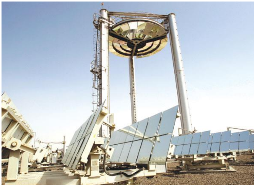
Figure 2-6 Masdar beam down plant [70]
