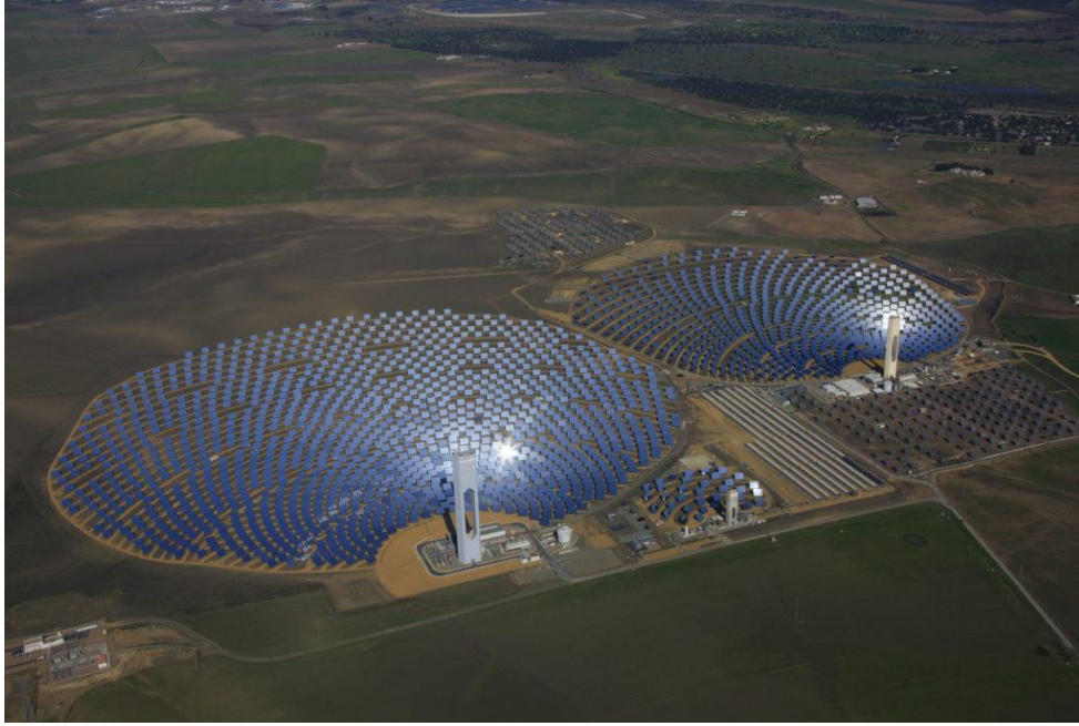
Figure 2-5 PS10 and PS20 power plant with cavity receiver (Source: Stela World)
