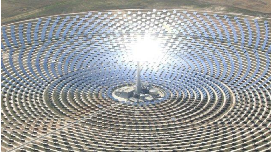
Figure 2-4 Gemasolar 20MW plant in Seville with an external cylinder receiver, Spain [67]
